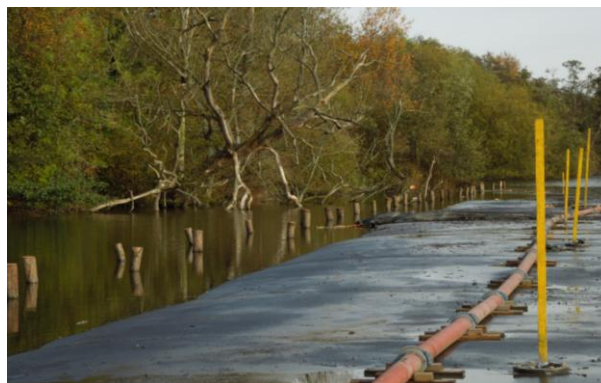
Figure 6. Gauging rods placed into the geotextile tubes.
