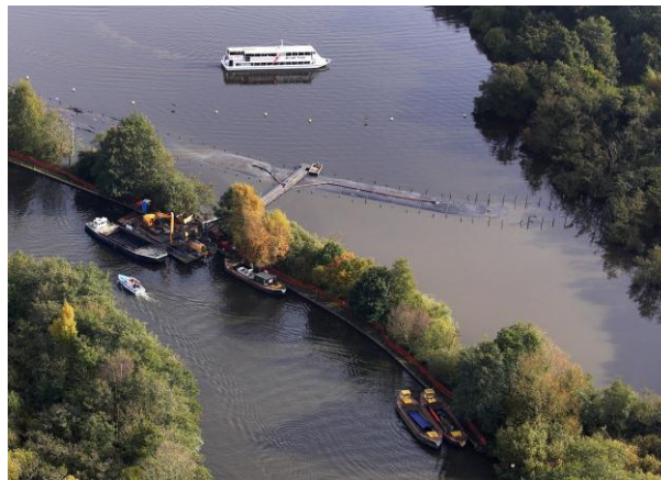
Figure 8. Filling of the geotextile tubes underway, November 2012 (Mike Page).
