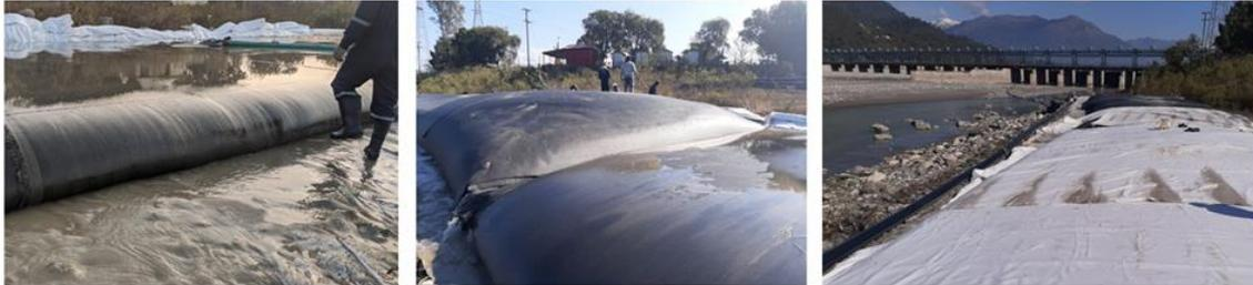
Figure 12 Geotextile tube along the eroded bank, downstream of the barrage.
